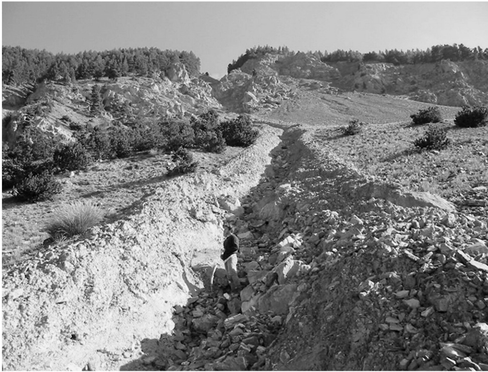
Fig. 6. Morphology of the eroded channel after the 2003 debris flow event at the Champerousse talus deposit in the upper part of the Faucon torrent.
